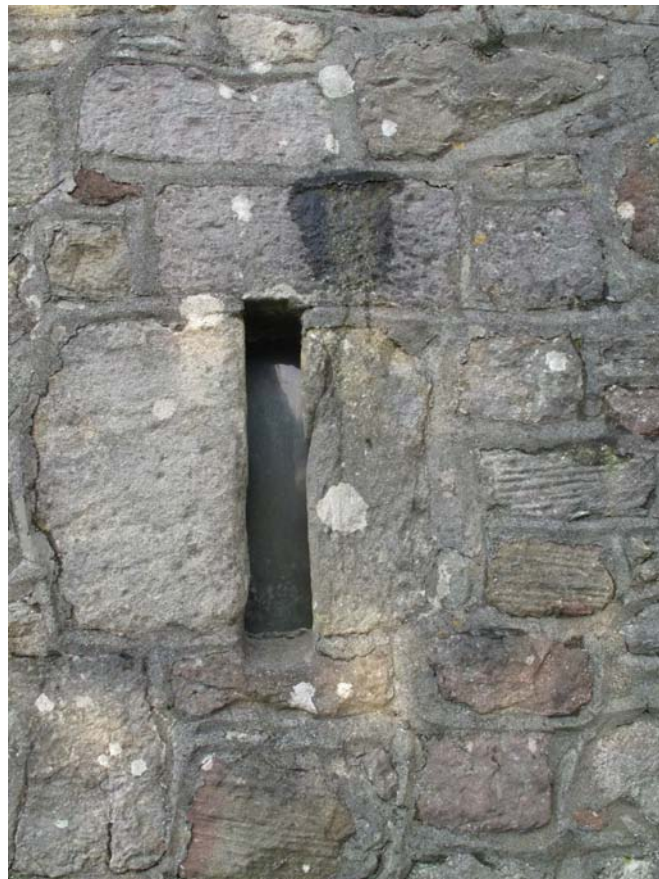
Fig. 10 – South window to mural stair with fixed glazing and profiled overpointing.
