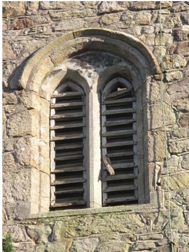
Fig. 12 – Condition of the west oak bell louvres showing their condition and poor fit to the surround.
