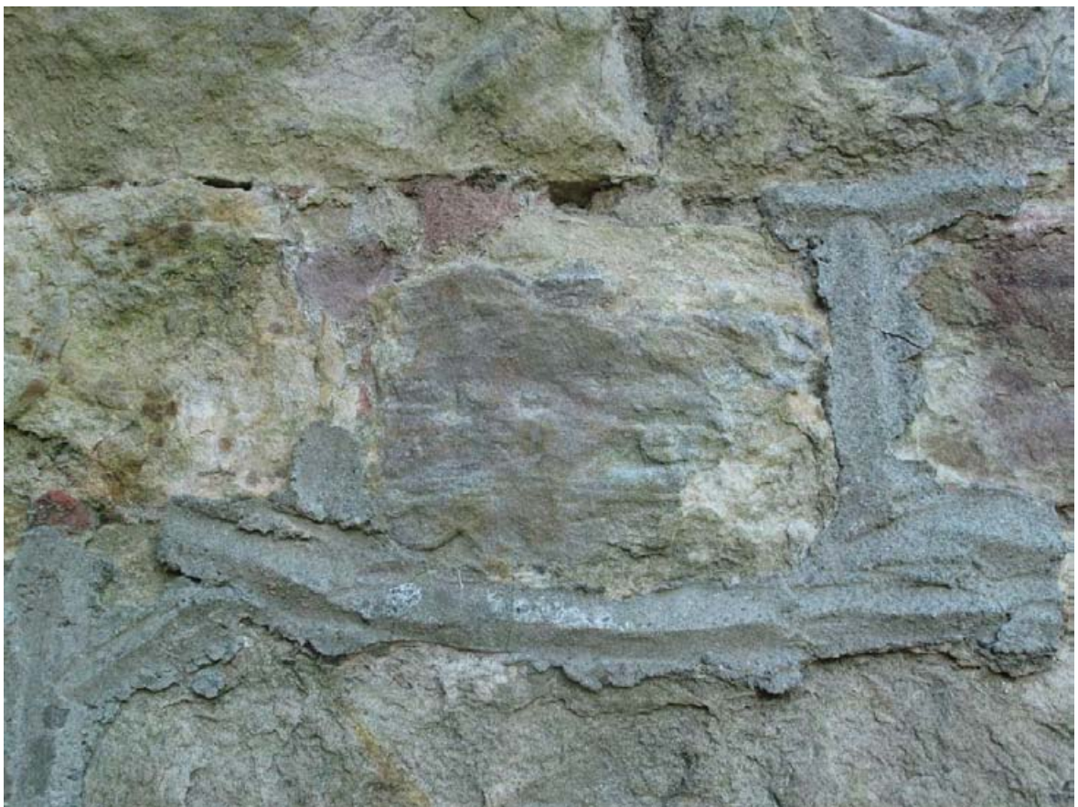
Fig. 18 – Superficial modern cement pointing on north wall over C19 mortar repairs showing the flush nature of the old joints
