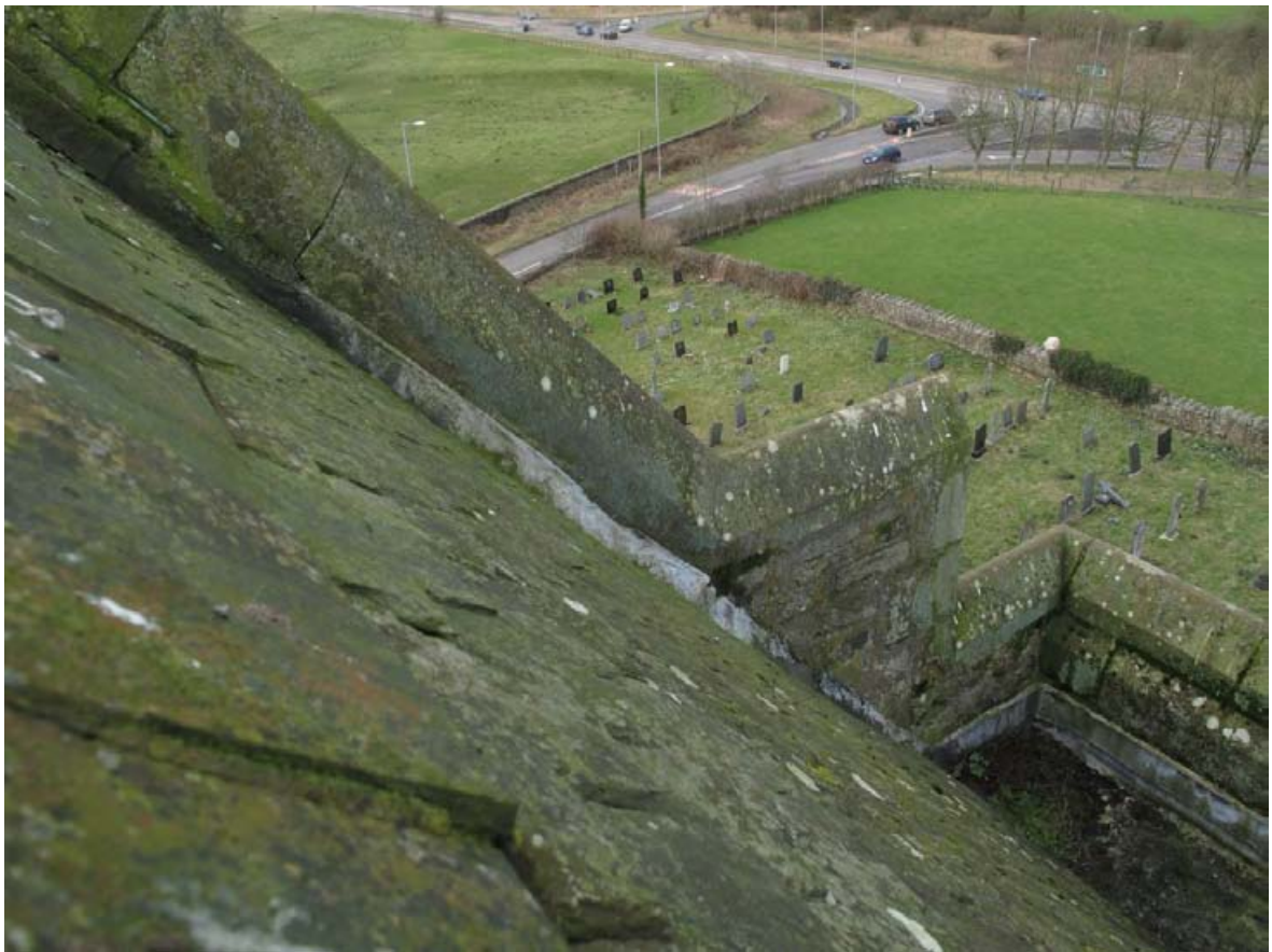
Fig. 25 - The north parapet gutter west flashings, copings and blocked gutter.
