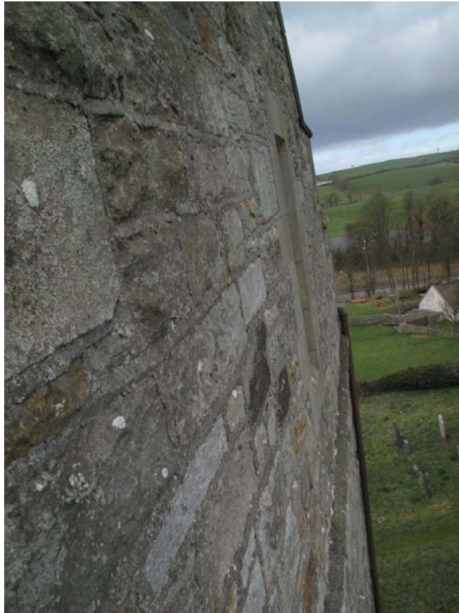
Fig. 21 - Loose pointing and open joints to upper stages of west wall.
