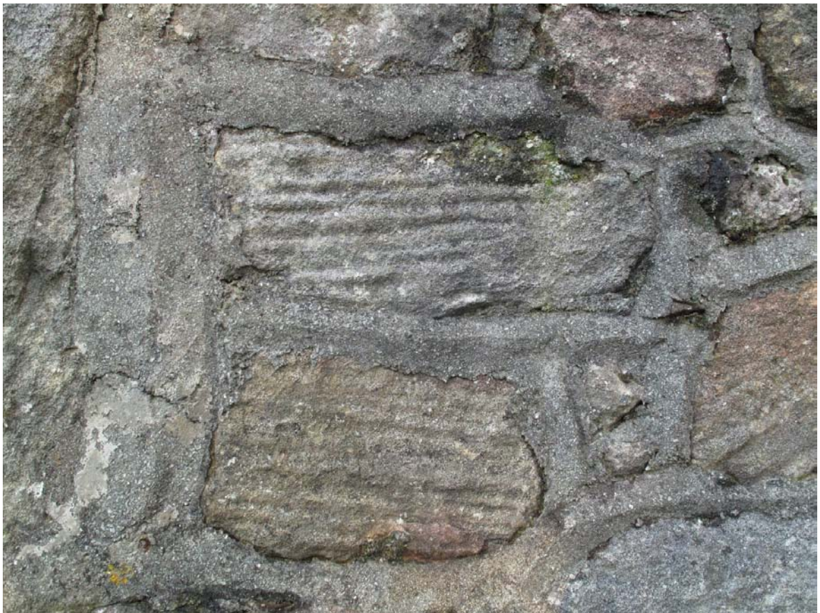
Fig. 17 – Condition of the south wall pointing with evidence of previous render.
