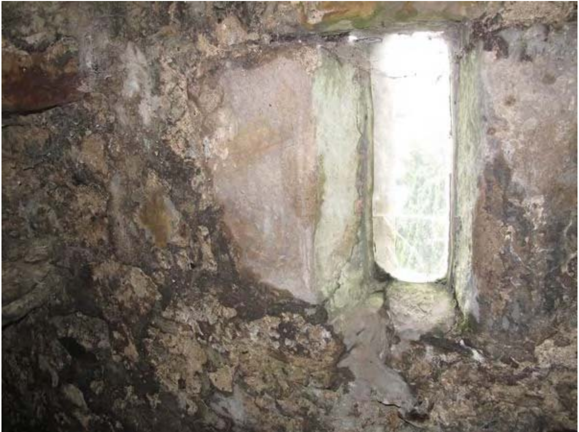
Fig. 33 – Fixed glazing to upper slit window with cement and mastic repairs.
