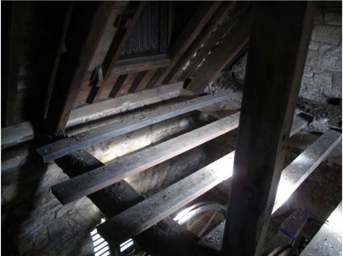
Fig. 36 – Inadequate access provision at roof level.
