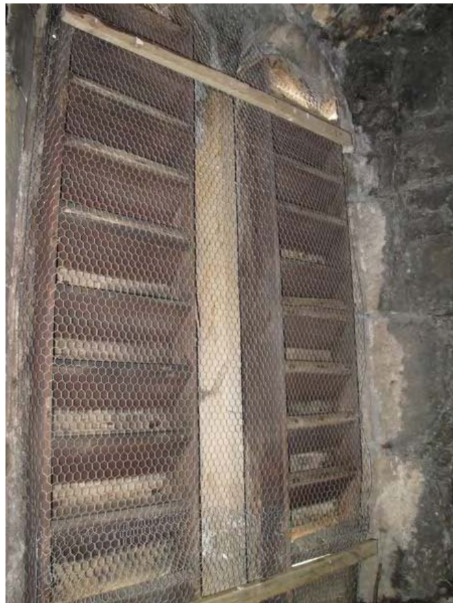
Fig. 34 – Condition of Belfry louvres and bird guarding.
