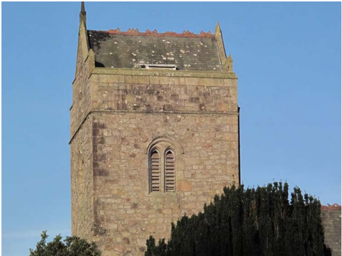
Fig. 5 – South parapet, slated roof and dormer roof access hatch.
