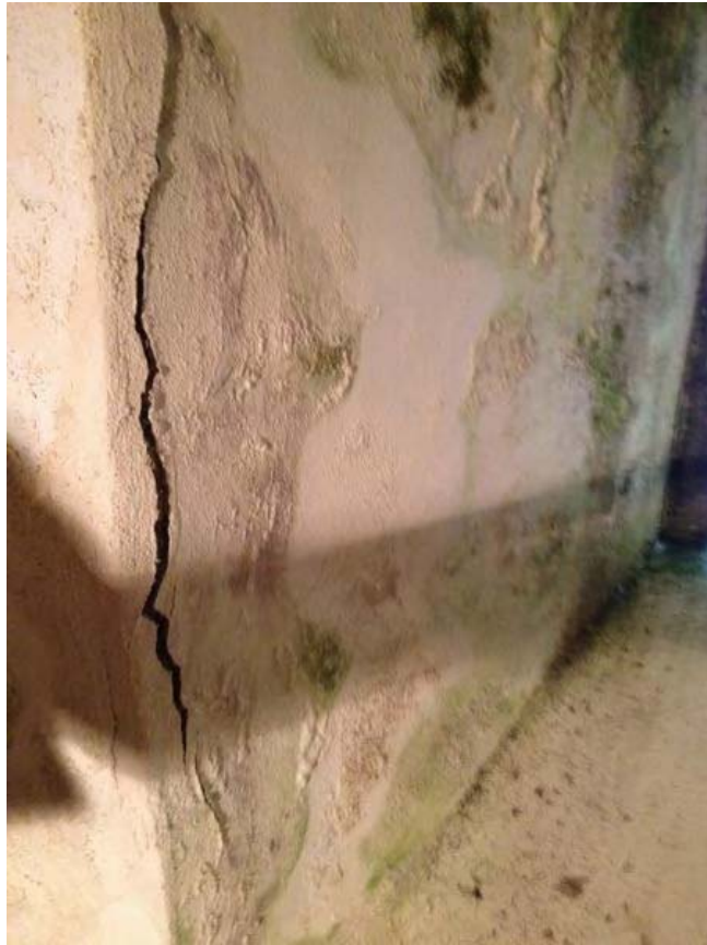
Fig. 31 – Plaster coats de-bonding from backing masonry due to high moisture levels and incorrect specification.
