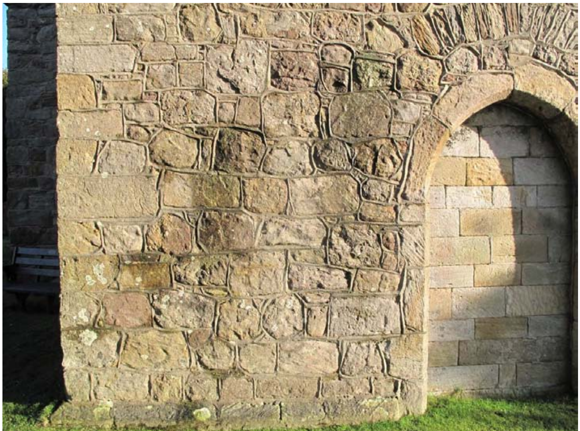
Fig. 14 – Blocked west door and surrounding projecting pointing and damp patches.
