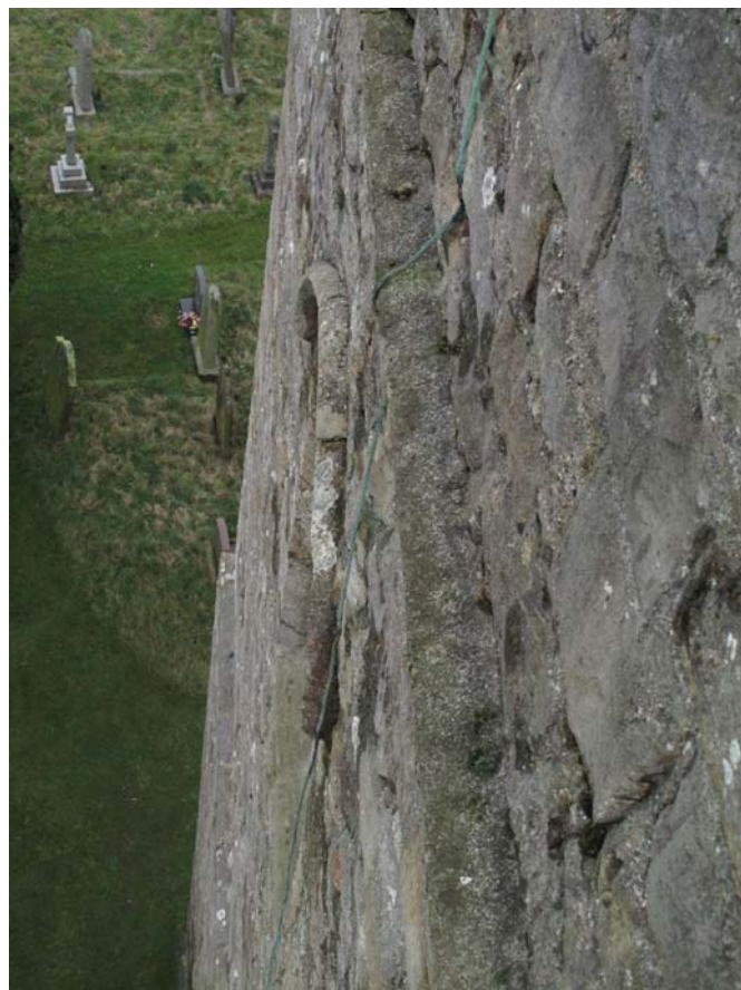
Fig. 20 – West wall scarpment with failing pointing and cement filet.
