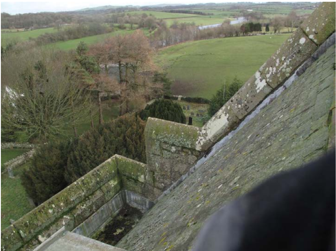
Fig. 24 – The north parapet gutter east flashings, copings and parapets.
