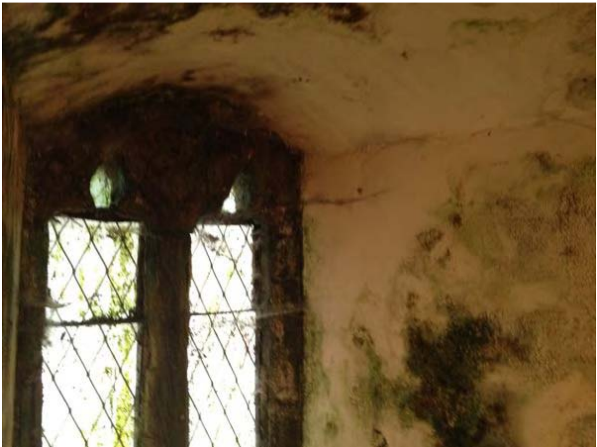
Fig. 29 – Damp conditions to window reveal and plaster failure.
