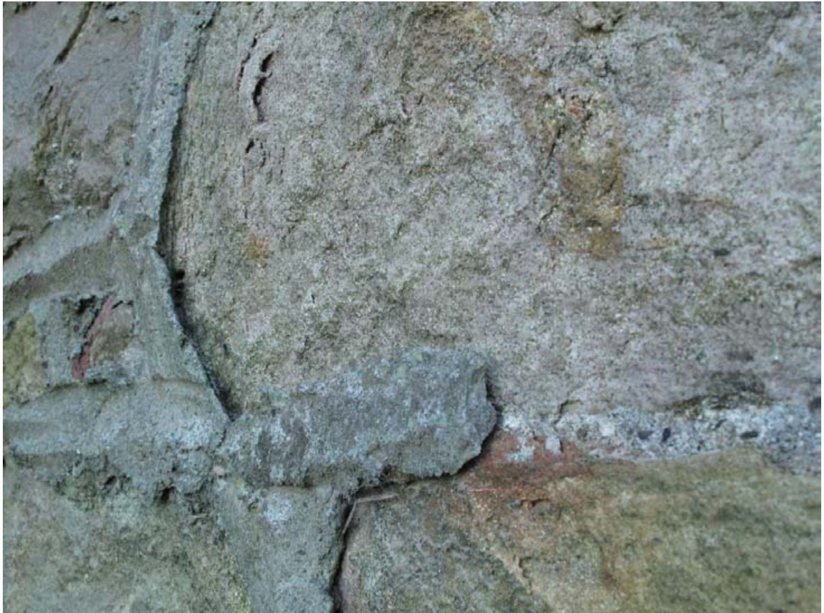
Fig. 19 – Failure of mortar joints over extant, flush lime mortar bedding.
