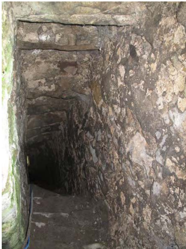
Fig. 32 – The mural staircase in the south-west corner with failed plaster finishes and water ingress through the outer walls and soffit.
