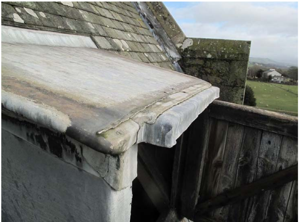
Fig. 26 – Condition of the south access dormer leadwork and patched leadwork flashings to copings.
