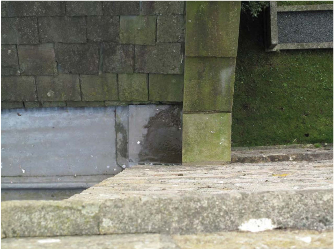
Fig. 23 – View of the abutment with the South Aisle gutter with pooling at the west end
