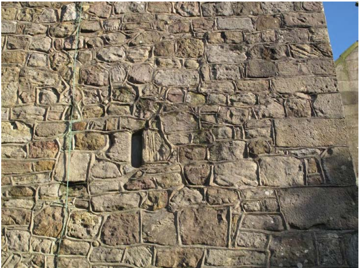
Fig. 15 – West window to mural stair with out-dated and inadequate lightning protection.
