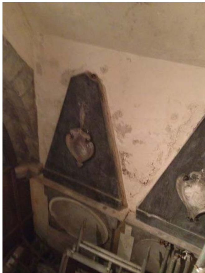
Fig. 30 – Plaster failure to ground floor surfaces and monuments.
