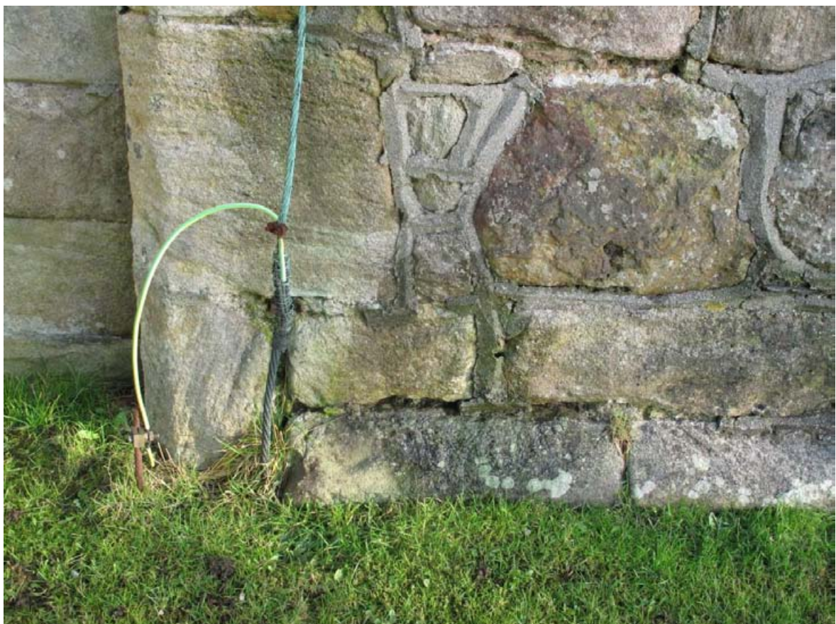
Fig. 16 – Open joints to base of wall and condition of failing cement pointing.
