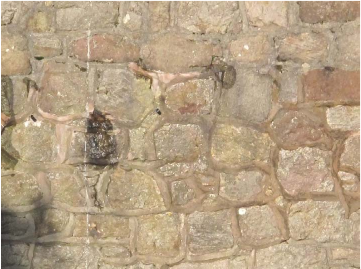
Fig. 11 – Condition of the pointing with water drying out from reservoirs within the wall core.
