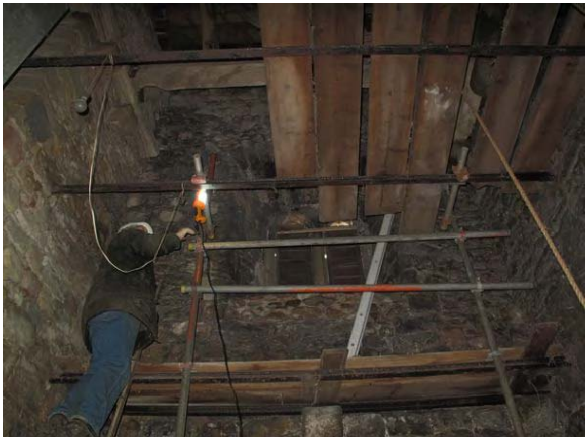
Fig. 37 – Access ladders and temporary platform at Belfry level.
