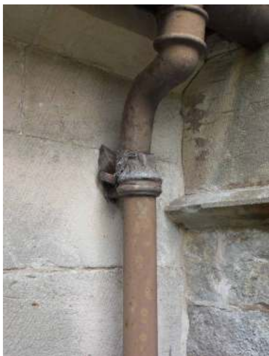
Figures 15 and 16: Detail of damaged downpipe to south porch (left) and overflow pipe in the north wall of the vestry, with iron corrosion staining to wall beneath (right).
