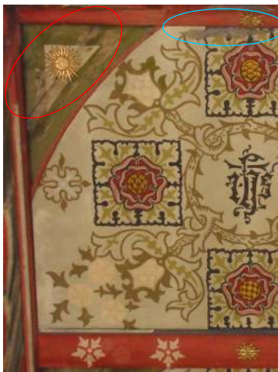
Figure 25: Detail of ceiling panel to north side of the ceiling showing cobwebs (blue circle) and evidence of water ingress, including staining and paint loss (red circle).
