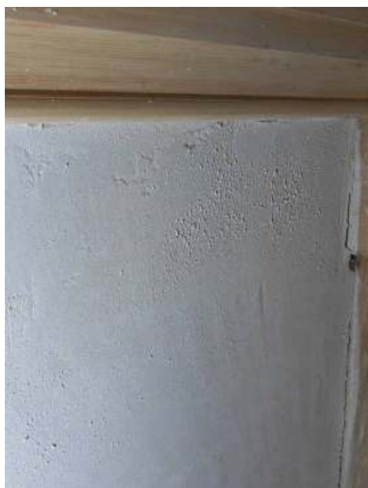
Figure 24: Detail of replacement plaster surface, showing uneven finish.
