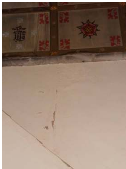
Figures 32 and 33: Detail of water damage to north westernmost panels, showing staining (possibly black mould), water run-off marks and disrupted wall plaster and paint beneath (right).
