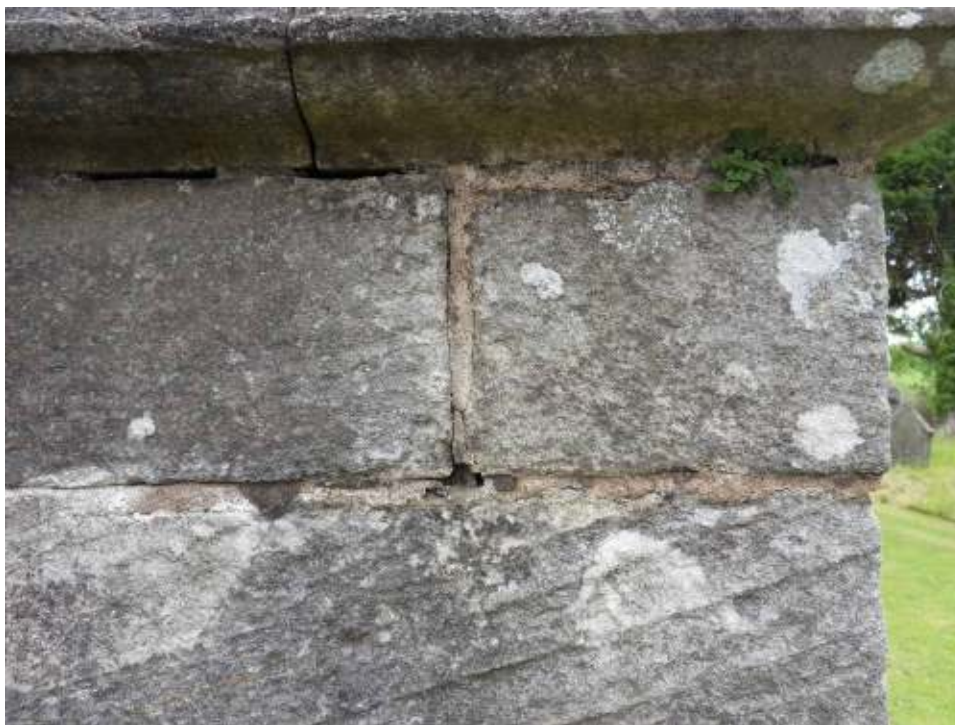
Figure 17: Detail of area of failing pointing on the south porch, with small plant growing out of void.
