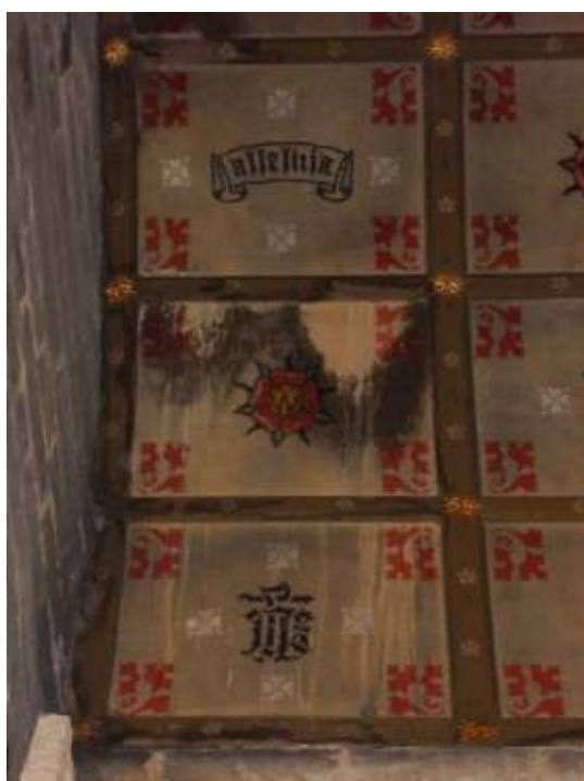
Figures 32 and 33: Detail of water damage to north westernmost panels, showing staining (possibly black mould), water run-off marks and disrupted wall plaster and paint beneath (right).
