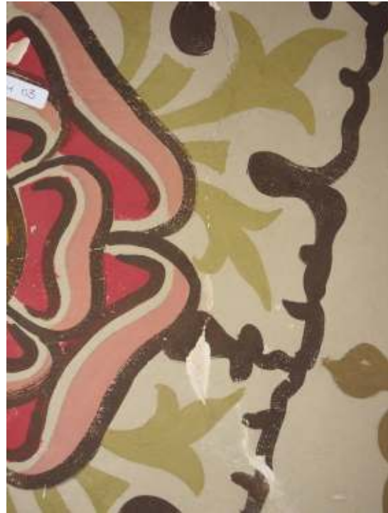
Figure 29: Detail of paint losses along the edge of a fine fracture.
