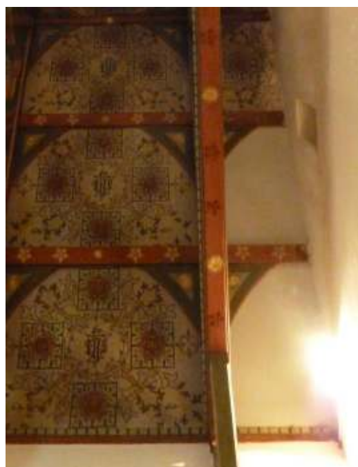
Figure 20: Detail of replaced plaster to two westernmost panels on south side of the ceiling. Note the water damage to the right side of the panel above.
