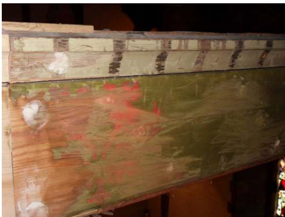
Figure 27: Detail of area of damage to original decoration following the fixing of replacement timber.
