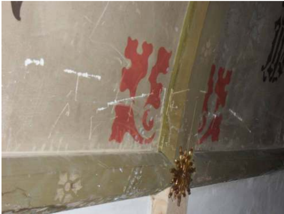
Figure 37: Detail of areas of impact damage – scratches and paint loss; these appear to be recent as there are no dirt deposits on the exposed plaster. Water staining and plaster marks can also be seen on the lower timber frame.
