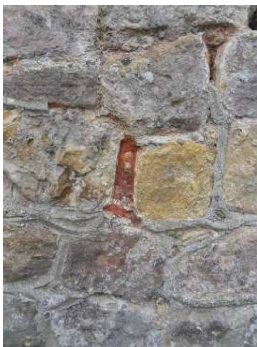
Figures 12 and 13: Details of extensive repointing to tower, west face (left) and north face (right).
