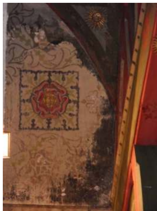
Figure 21: Detail of water damage and staining (possibly mould) to lower westernmost panel on north side of the ceiling. Access to this panel was not available on the day of the inspection.
