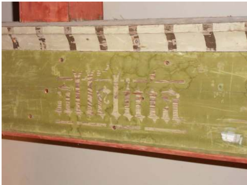
Figure 30: Detail of timber beam showing unfilled fixing holes and paint losses, particularly evident in the text following the grain of the wood.
