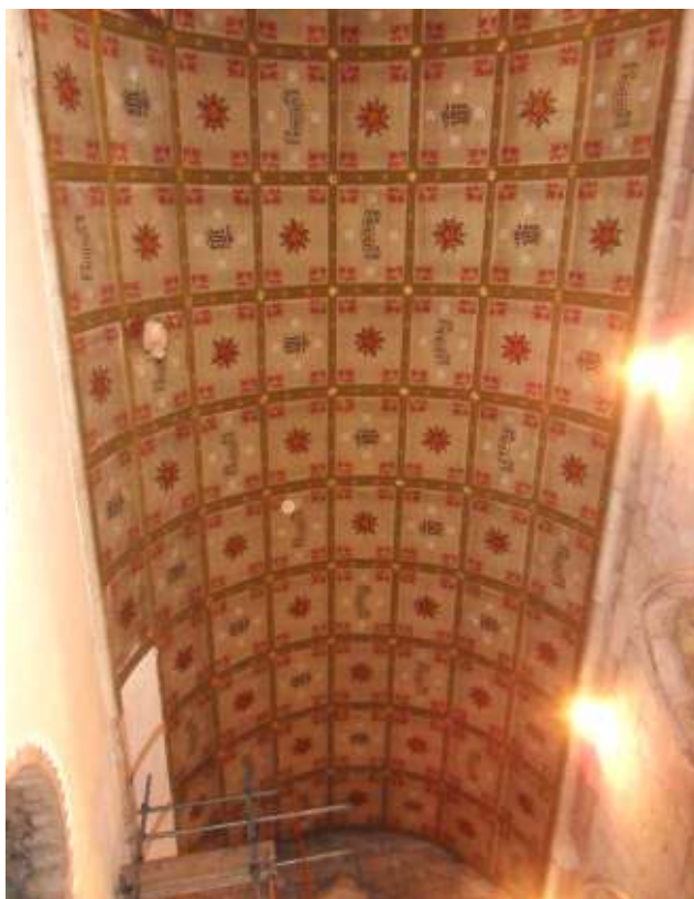
Figure 31: Overview of the south aisle ceiling. Note the replaced plaster panels in the north east corner, with access scaffold beneath.
