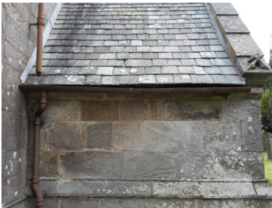
Figure 14: Guttering to west side of south porch, showing deformation and slight split.
