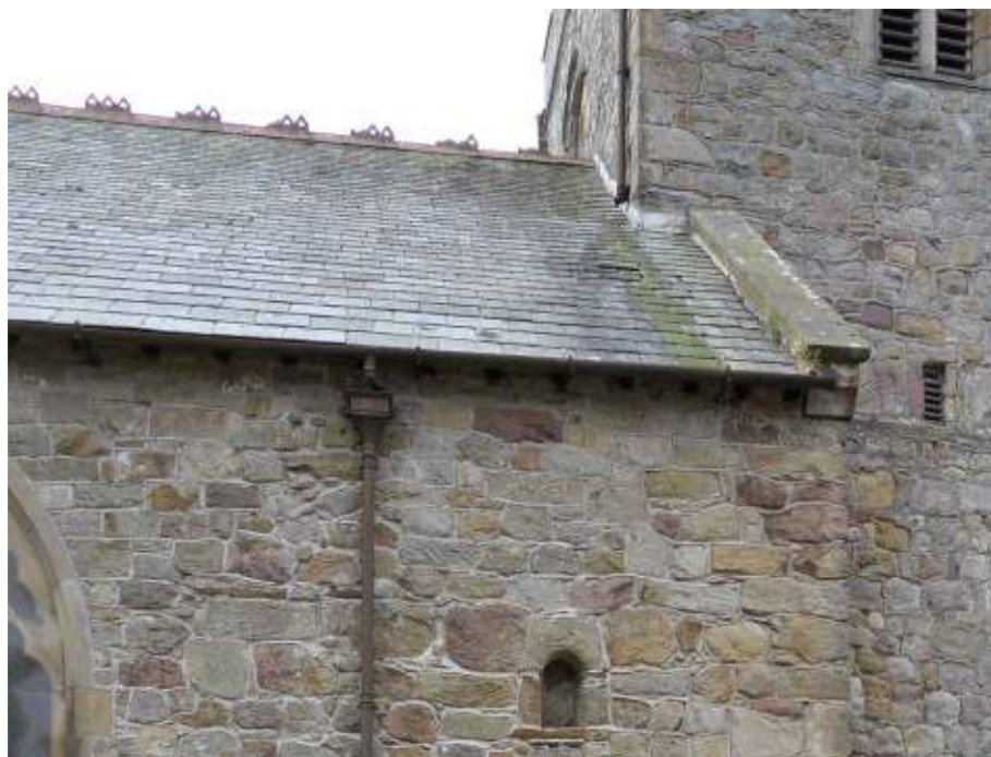
Figure 11. Detail of north-west corner of nave roof, showing lost detailing to ridge tiles, cement flashing, mildew and grass growth.
