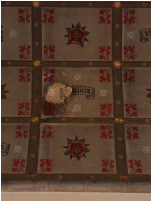
Figure 34: Detail of staining and water run-off marks as a result of historic water ingress.
