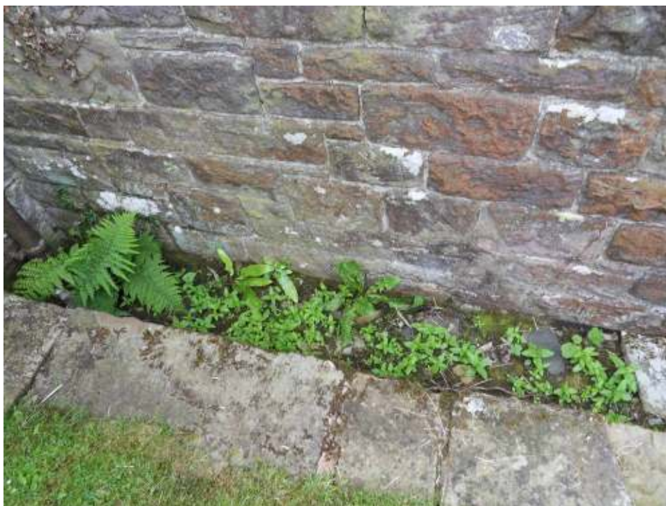
Figure 18: Extensive biological growth found in the north gully.
