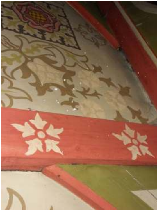
Figure 28: Detail of ceiling panel to south side showing white splashes of plaster, presumably from the recent repairs.
