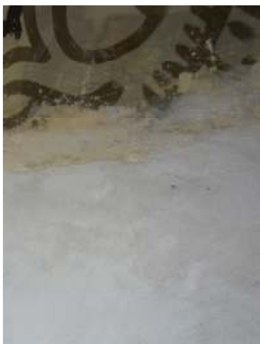
Figure 23: Detail of junction between replacement plaster and original decoration. Note the uneven finish and step in plaster edge.
