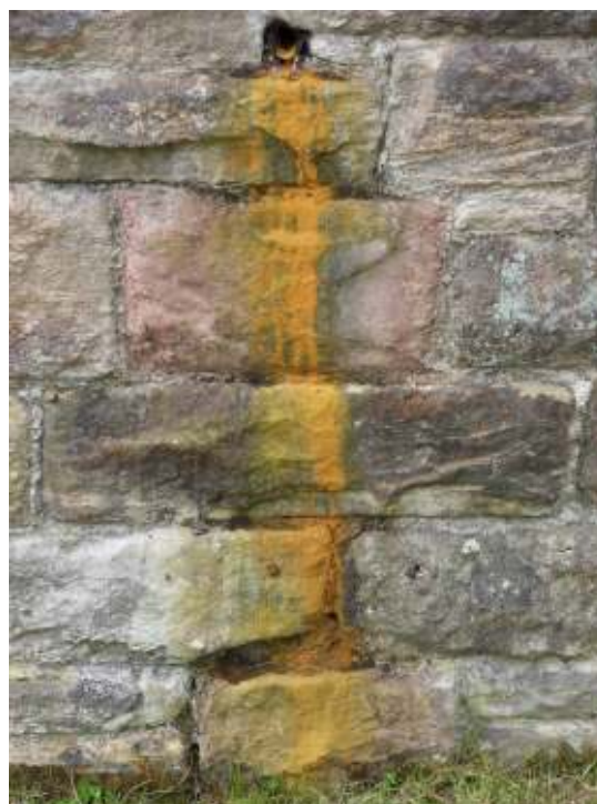
Figures 15 and 16: Detail of damaged downpipe to south porch (left) and overflow pipe in the north wall of the vestry, with iron corrosion staining to wall beneath (right).
