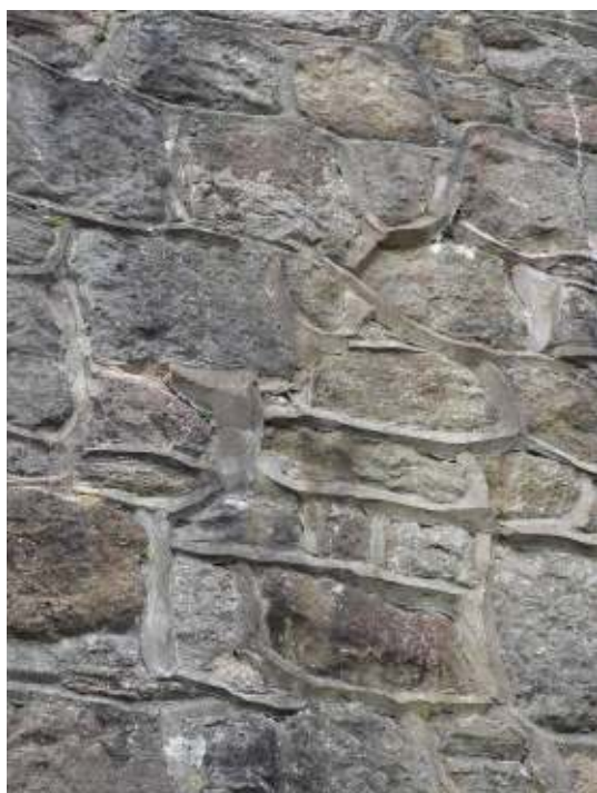
Figures 12 and 13: Details of extensive repointing to tower, west face (left) and north face (right).
