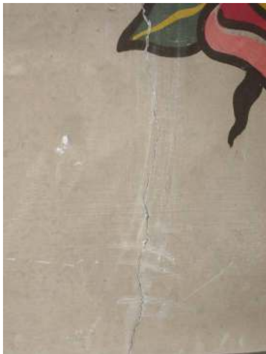
Figure 38: Detail of fine fracture in surface of panel, with minor areas of flaking paint along its edge.
