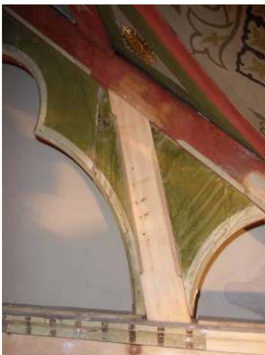
Figure 26: Detail of replacement timber and water run-off marks and lost paint to original decoration.
