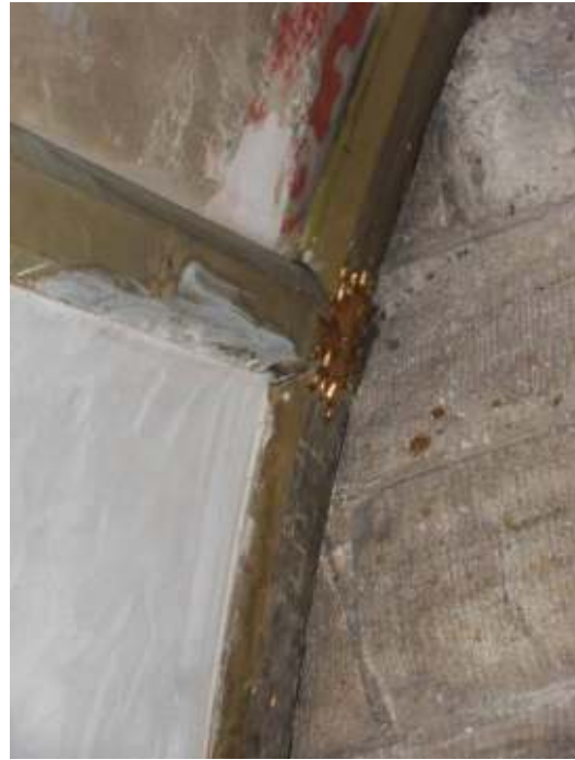
Figure 35: Detail of area of replacement plaster, showing staining to original decoration of surrounding timber frame.
