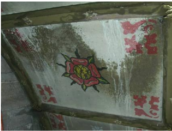
Figures 30 and 31. Details of water stained and salt damaged panel before (left) and after (right) treatment.
