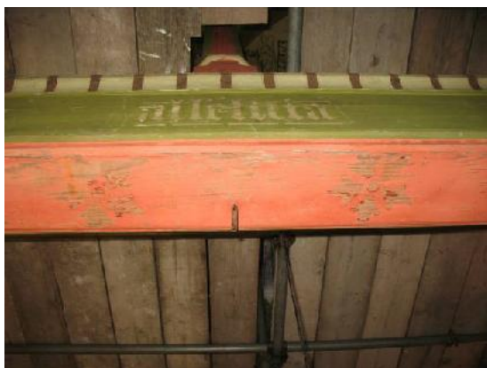
Figures 12 and 13. Details of the underside of a beam before and after recreation of missing stencilled design.
