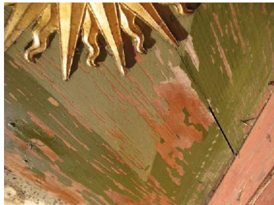
Figures 6 and 7. Details of an area of flaking paint before (left) and after (right) the spray application of consolidant.
