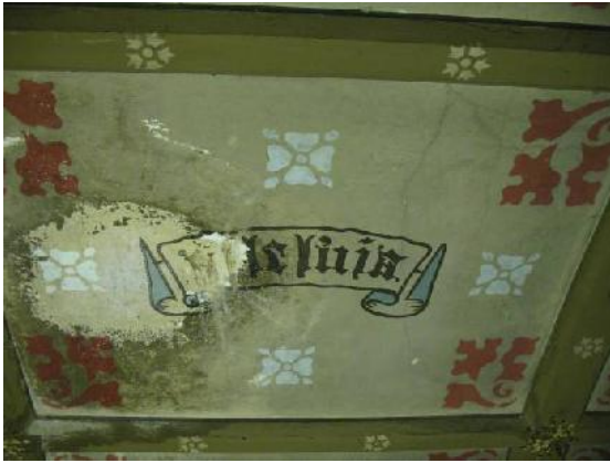
Figures 28 and 29. Details of water stained and salt damaged panel before (left) and after (right) treatment.
