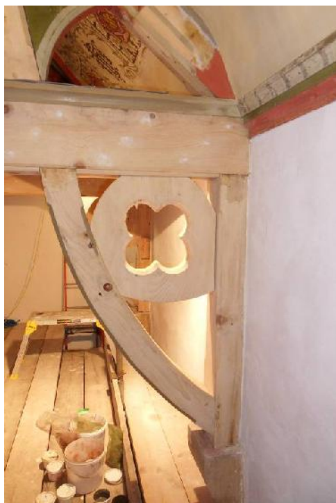
Figures 14 and 15. Details of replacement beam and truss before and after recreation of decoration.
