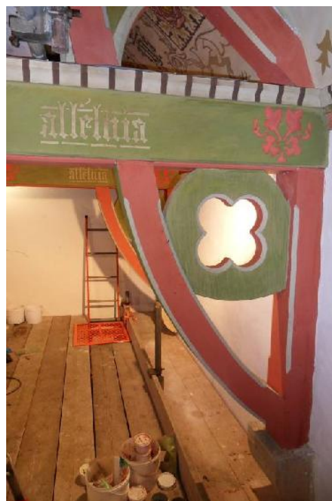
Figures 14 and 15. Details of replacement beam and truss before and after recreation of decoration.
