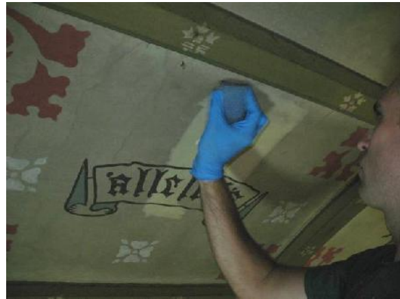
Figures 23 and 24. Detail of injection of consolidant behind loose paint flake (left), and dry cleaning the painted panels using Wishab sponge (right).
