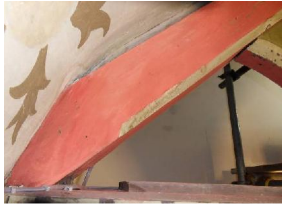
Figures 19 and 20. Details of area of tide marks/water staining before and after toning with dry pastels.
