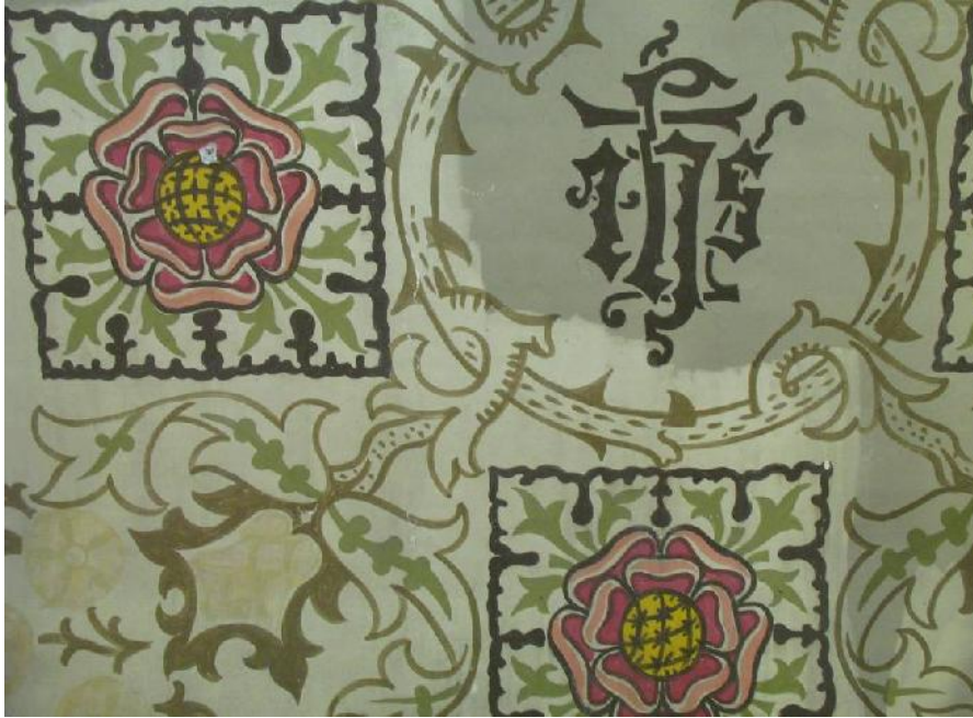
Figure 8. Detail of ceiling panel during cleaning with a Wishab sponge.
