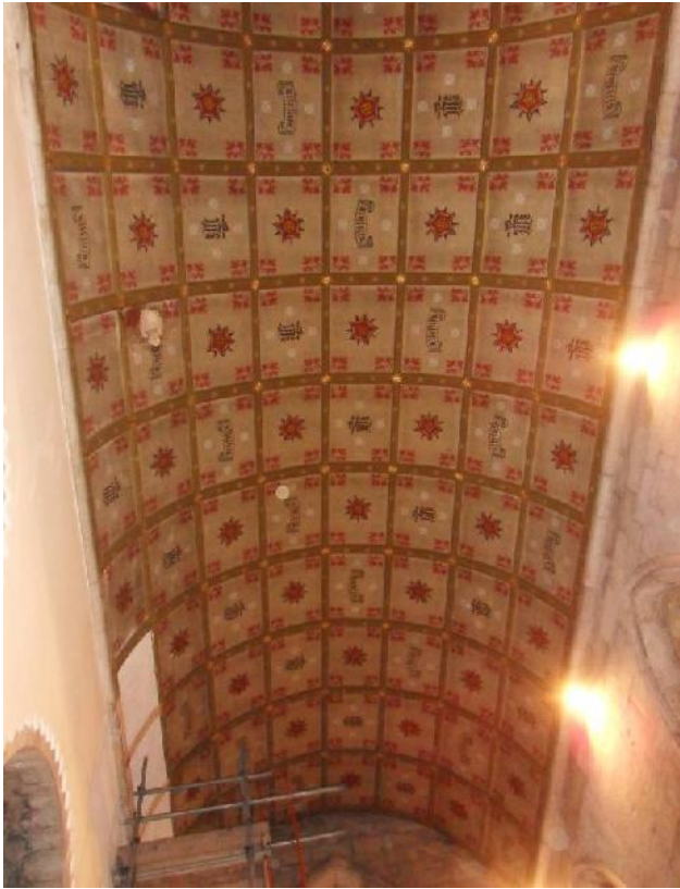
Figure 22: Overview of the south aisle ceiling during the condition assessment. Note the replaced plaster panels in the north east corner, with access scaffold beneath.
