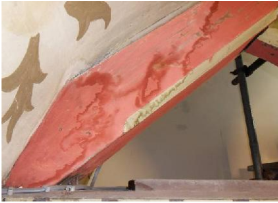
Figures 19 and 20. Details of area of tide marks/water staining before and after toning with dry pastels.
