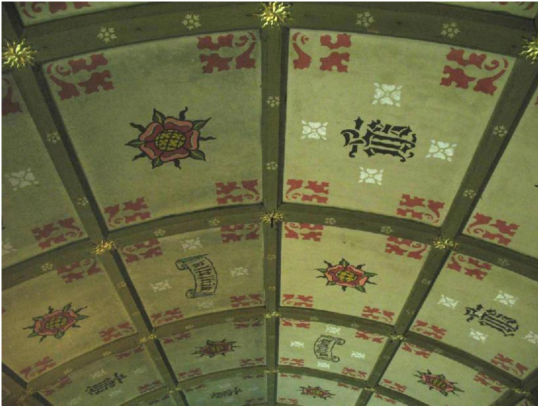
Figure 25. Section of the ceiling during cleaning – note the cleaned panels on the right hand side.
