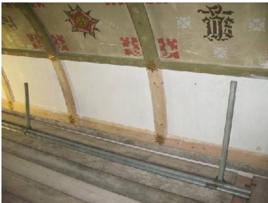
Figures 32 and 33. Details of replaced plaster panels in north east corner before and after recreation of stencilled decoration.
