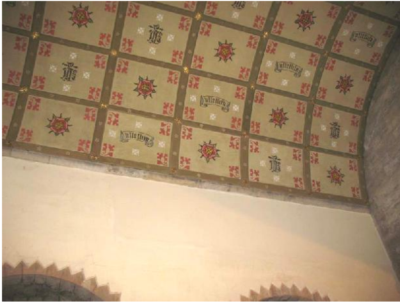
Figure 34. Overview of north east corner panels and colour matched distemper to upper wall following removal of scaffolding.
