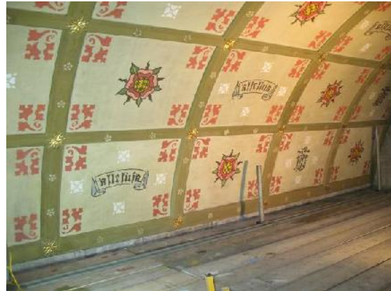
Figures 32 and 33. Details of replaced plaster panels in north east corner before and after recreation of stencilled decoration.
