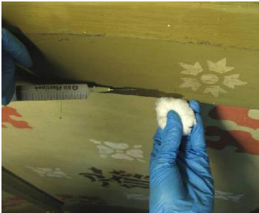
Figures 23 and 24. Detail of injection of consolidant behind loose paint flake (left), and dry cleaning the painted panels using Wishab sponge (right).
