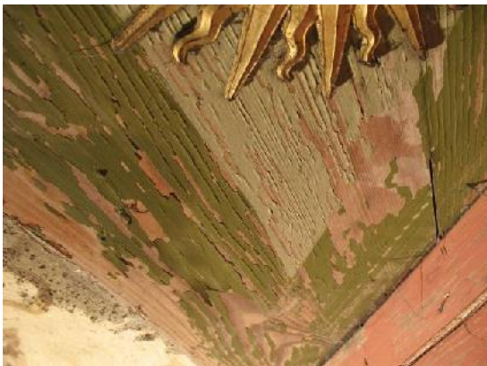
Figures 6 and 7. Details of an area of flaking paint before (left) and after (right) the spray application of consolidant.
